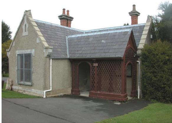
*Figure 1 The Sexton's Cottage, Northern Cemetery. PVC down pipes and unsympathetic mesh screen over window detract from aesthetic qualities of this heritage-listed building. (Photo: C Betteridge, April 2004)*
